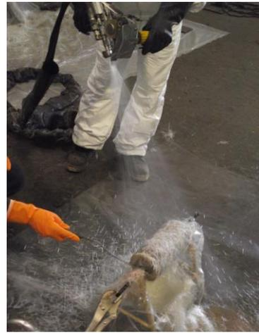
Figure 2: SGFRP strengthening process
