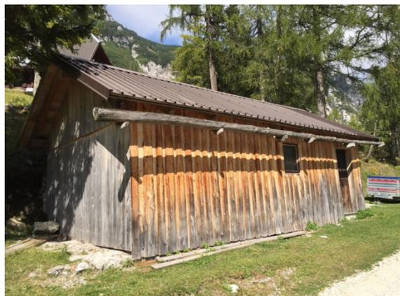
**Figure 1:** Figure illustrating the undesired uneven discoloration of wooden façade exposed to an outside environment: an adequate protective anti-UV coating limits the weathering effects that can then lead to deterioration of wood.
